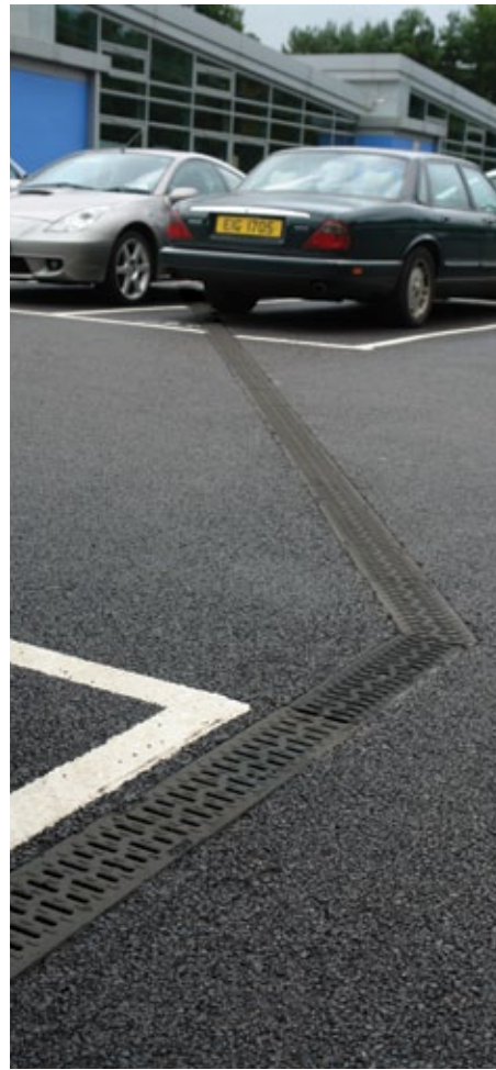
ACO ParkDrain, a monocast channel drainage system was used in a number of areas throughout the school to provide a sustainable drainage system.
