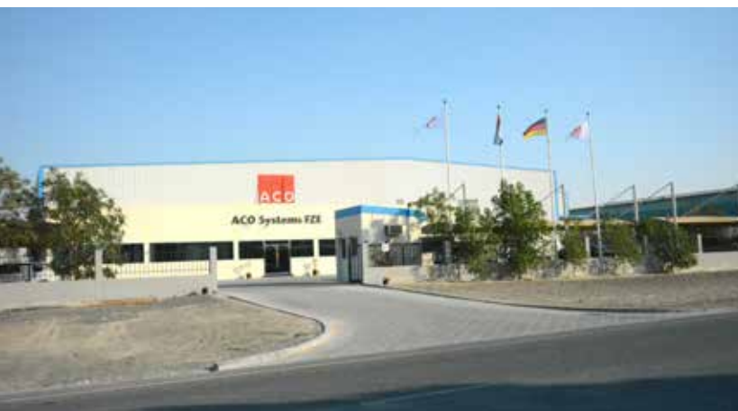
ACO Systems FZE in Dubai, United Arab Emirates
