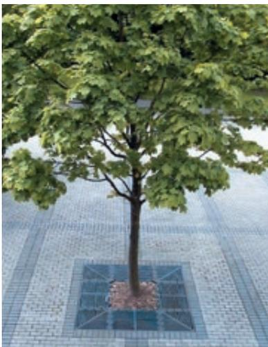
ACO Wotan tree gratings are variable in size and shape. A subsequent adaptation to suit the tree growth is also possible. With round, square or rectangular tree gratings as well as protective gratings in corners or on a wall, creative open space design is possible. And all this unsupported without substructure.
