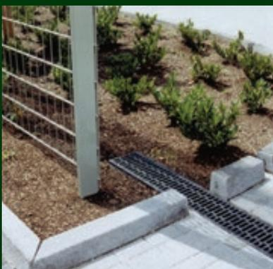
Drainage channels absorb the rainwater safely and direct it away close to the surface into the adjacent green area. There it can gradually seep away – and the plants and greenery are irrigated in a targeted manner.
