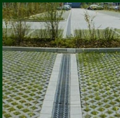
Permeable surface area coverings enable precipitation and rainwater to seep away directly from where it accumulates. During heavy rainfall and ground frost, precipitation and rainwater can be safely discharged through drainage channels.
