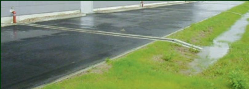
Drainage channels close to the surface discharge precipitation and rainwater quickly and easily into the infiltration troughs.
