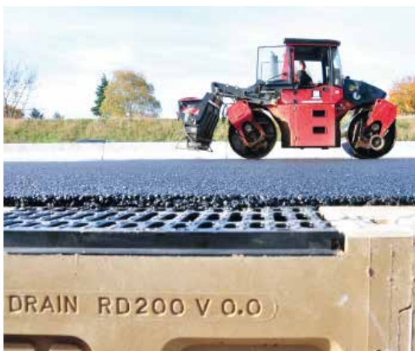
Drainage of porous asphalt
