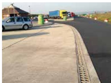
ACO DRAIN® Monoblock RD 200 V in a motorway service station
