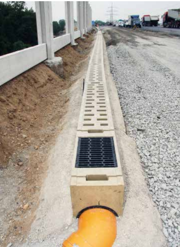
ACO DRAIN® Monoblock RD 300 during installation on the A3 motorway
