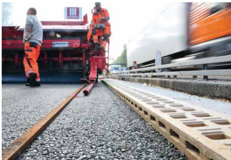
ACO DRAIN® Monoblock RD 200 V DF on the A1 motorway, Hamburg section
