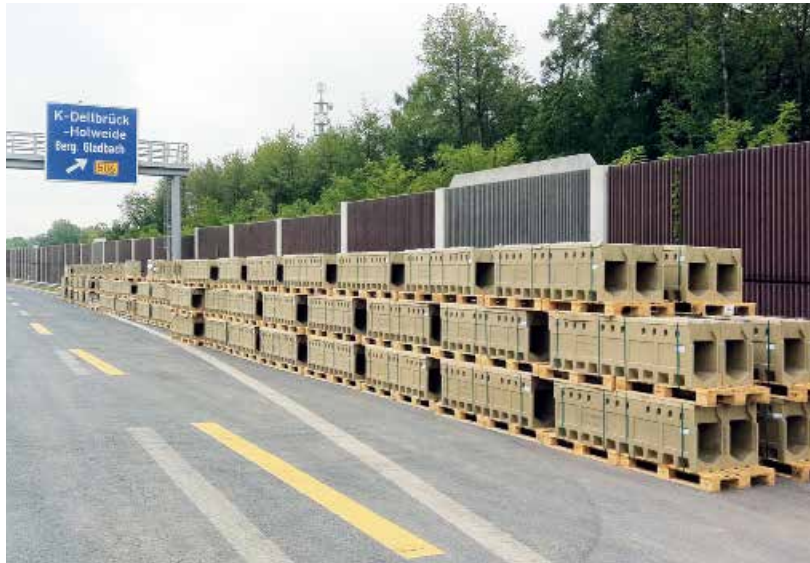
ACO DRAIN® Monoblock RD 300 DF for the widening of the A3
