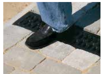
The grating is pressed on briefly to lock it
