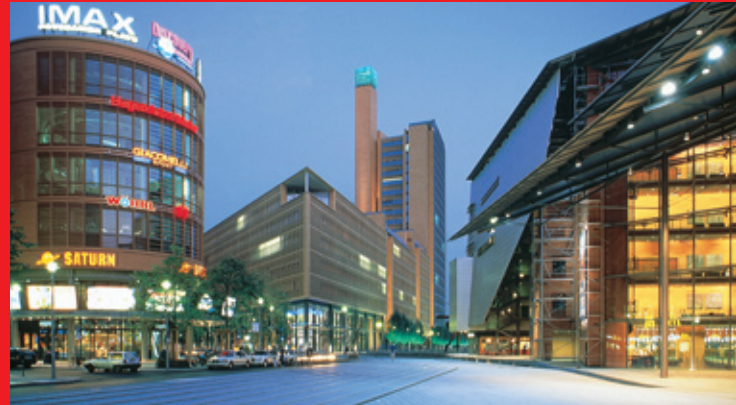
ACO surface drainage for Potsdamer Platz, Berlin
