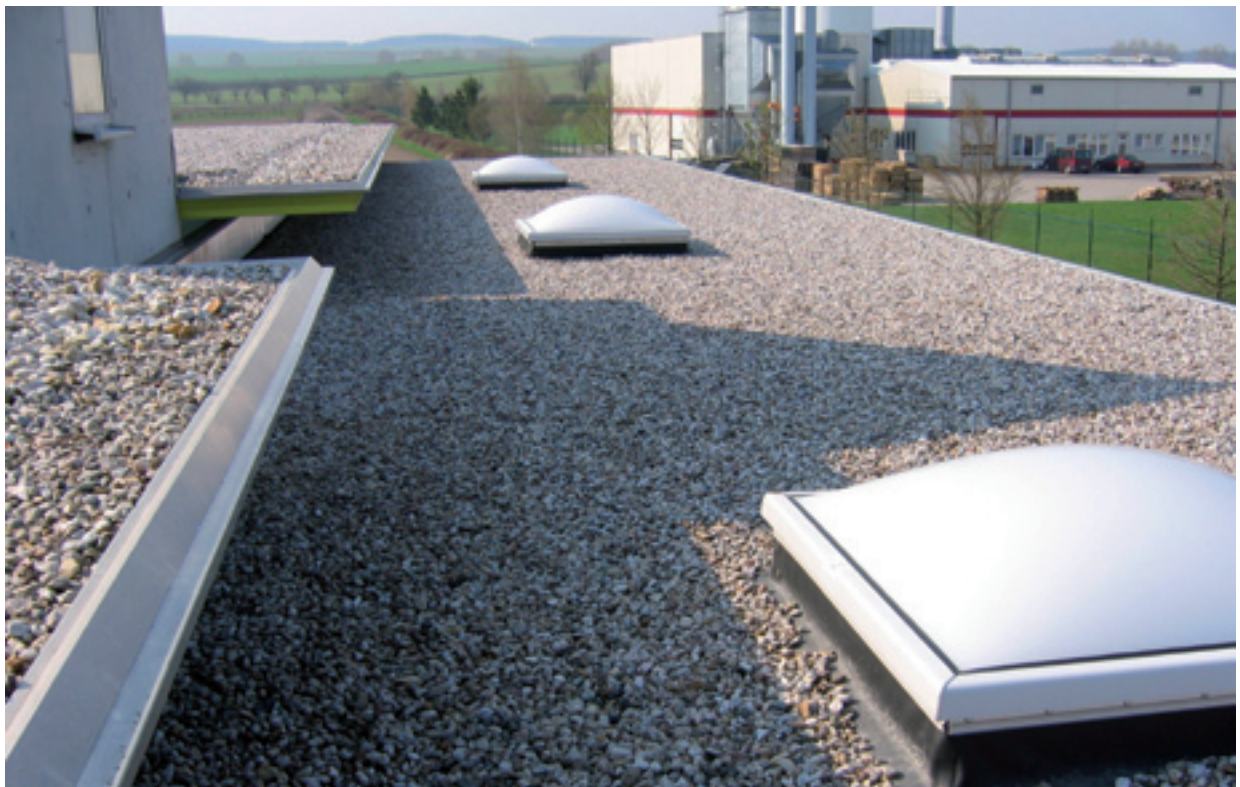
Flat roof with a gravel protection layer
