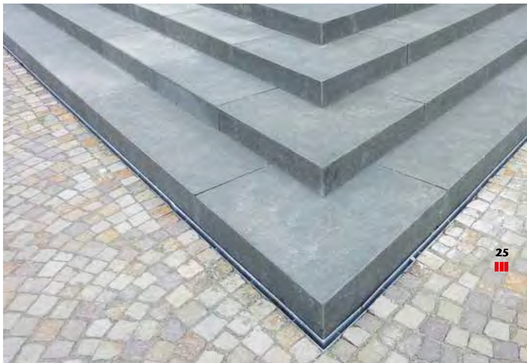
Steel slot channel Page 43
