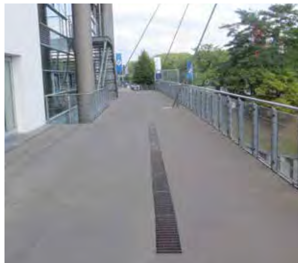
Stainless-steel channels for covered areas
