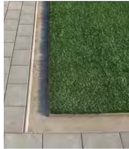
Trough channel for filled-pile artificial turf
