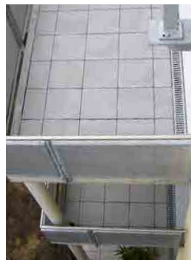
Open channel with drainage above the roof waterproofing membrane: balcony with the ACO Self® Highline
