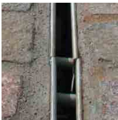
Slotted frames that abut each other without the connector clip
