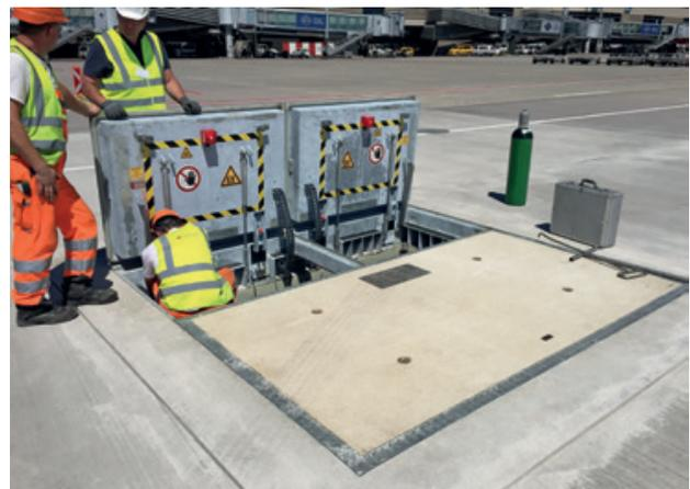
The ACO Servokat access covers are the ideal solution when covers have to be moved frequently for maintenance and inspection work. The covers with assisted-opening can be easily operated by one person. The surface covering integrated within the top is completely variable to ensure full incorporation within the design concept at each location.
