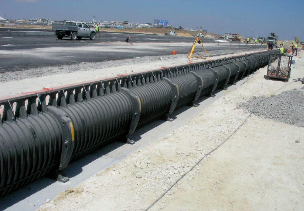
Alignment and start of installation of the Qmax 900 channels
