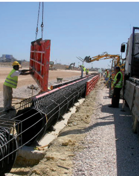
Site, installation of reinforcement and side formwork
