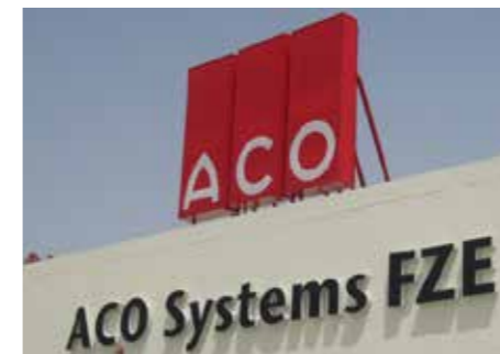
ACO Building Warehouse and offices
